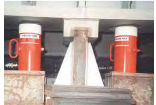
C10010C used in this lift application.
